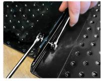
STEP THREE (Cont.): Attach the Cross-over Bridge to the Outside Ramp - Align the pre-drilled holes on the outdoor ramp and place the ramp through the bolts. Add another washer followed by the nut to each bolt. Use a wrench to hold the nuts in place while you tighten the bolts. Do not over-tighten bolts.
